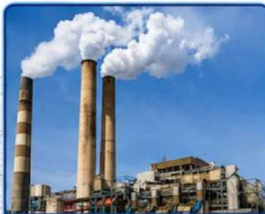
SLURRY & ASH HANDLING
